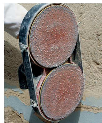
Removing old plasters
