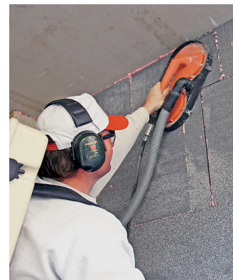
Grinding EIFS and ETICS boards
