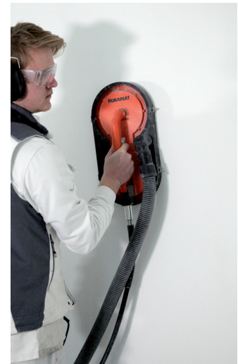
Grinding plaster
