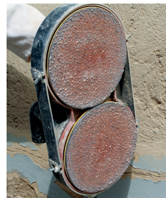
Removing old plasters
