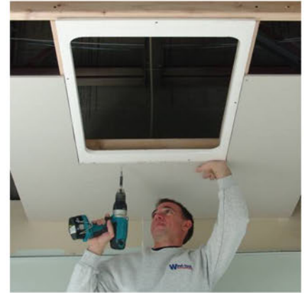
3. Hang drywall around the panel frame.
