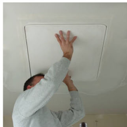
5. Once dry, smooth tape joints and install your panel door.
