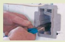
STEP 2: Insert the INEXO box into your opening and push the 'teeth' into place until you hear the 'click' – so you know your box is secure. If you are positioned next to a tie, you can utilize two of the 'teeth' on the non-tie side and use the flange holes on the opposite side to screw into the plastic tie.
