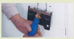
STEP 1: Select the position for your box. Using a hot-knife or cutting tool, cut the opening in the EPS foam.
